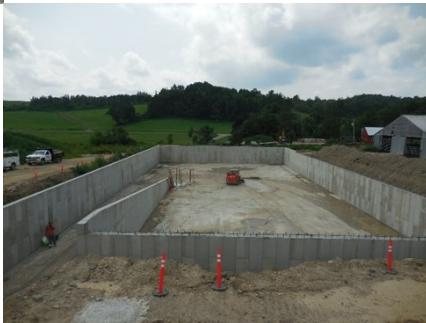
The walls were poured and removed to allow to cure before backfilling could start.
